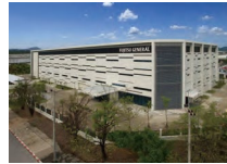
FUJITSU GENERAL AIR CONDITIONING R&D (THAILAND) CO., LTD.
