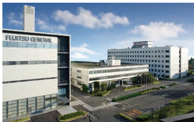
Fujitsu General Headquarters
