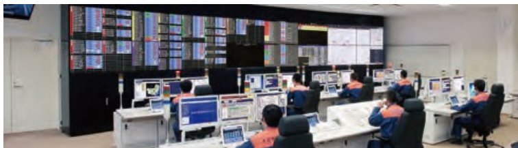
▲ High-performance firefighting command center
