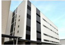
Kawasaki Headquarters/ Innovation & Communication Center
